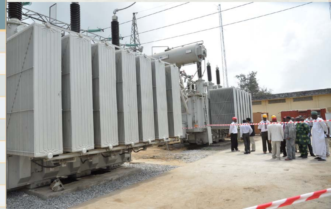
2x60MVA 132/33 transmission substation in ojo Lagos
