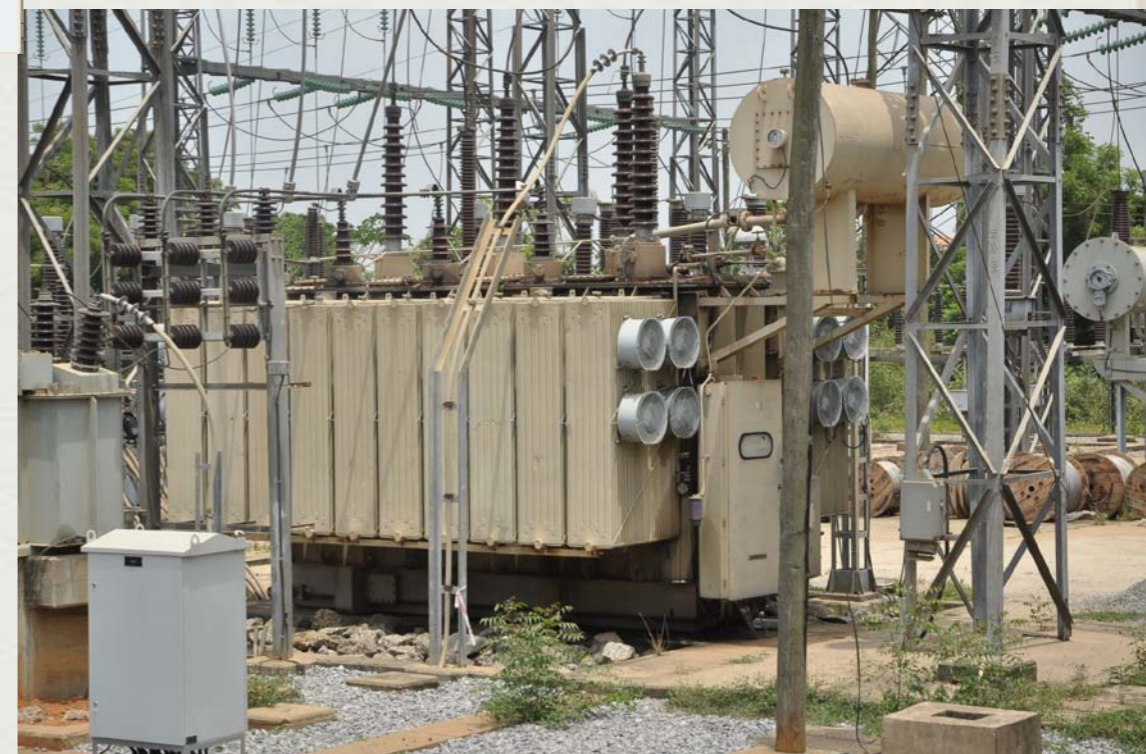
2x60MVA 132/33 transmission substation in ojo Lagos
