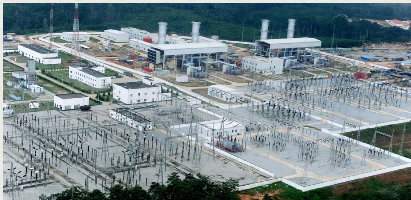
Omotosho 451 MW Power Plant
